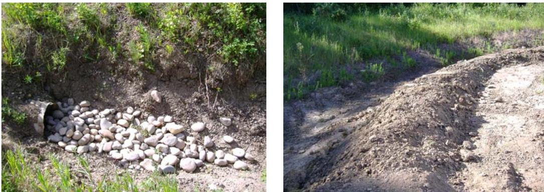
**Figure 3 – Culvert rip-rap and berm repairs to control water**
